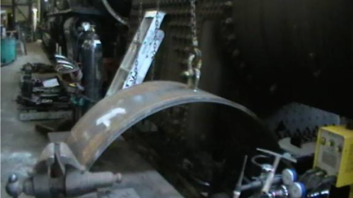
Patch plate rolled and ready to be lifted into position for fitting.
