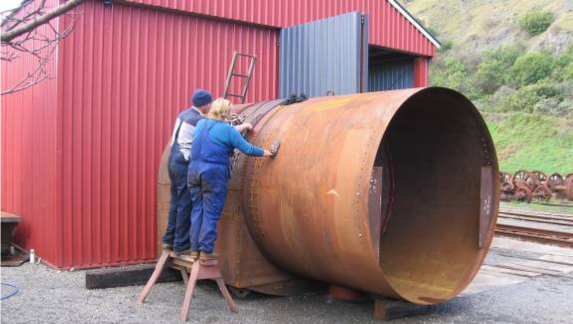
Peter Norman and Linn Alexander drill holes in one of the doubling plates for the tender body before Huck-bolting them in position. In this view, the front, bunker section of the tender body is upside down.
