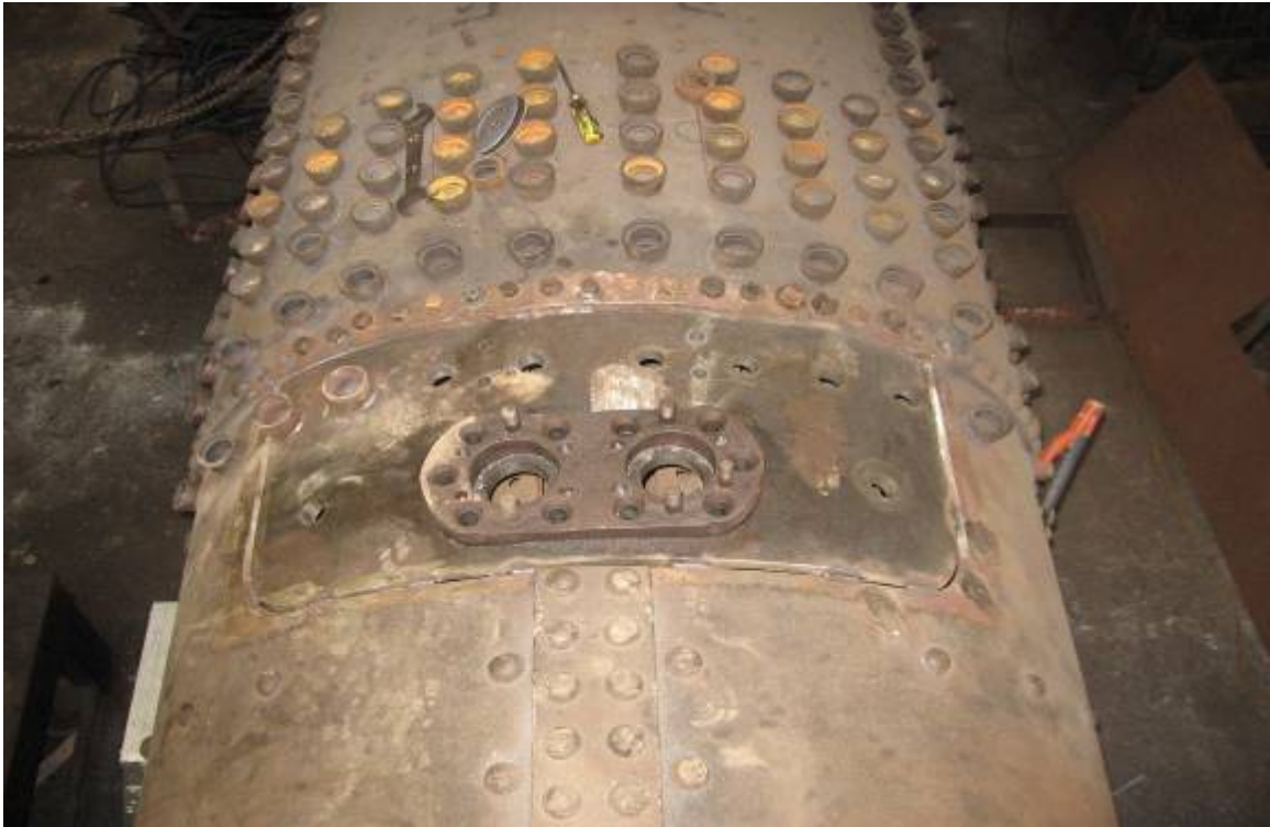
One of the patches required in the boiler of Ab 608 – This outer shell section includes the mountings for the safety valves.
