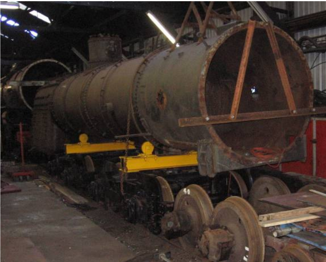
Ab 608's boiler mounted on roller-equipped accommodation bogies in preparation for major boiler repairs.
