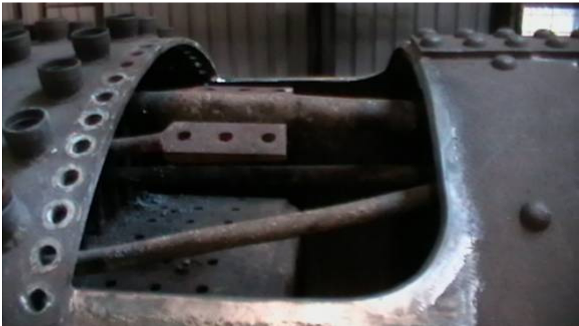
Boiler prepared to receive patch.
